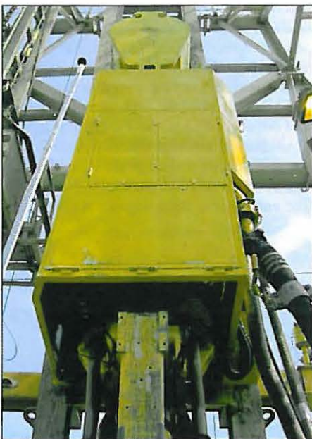
Fig. 4 Top drive with sound protection hood
